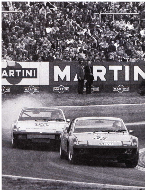
Ernst Strähle (foreground) does battle with one of the Max Moritz cars. An example of the wide variation in 914/6 GT models, the Moritz car has a roll bar while the Strähle car does not.
